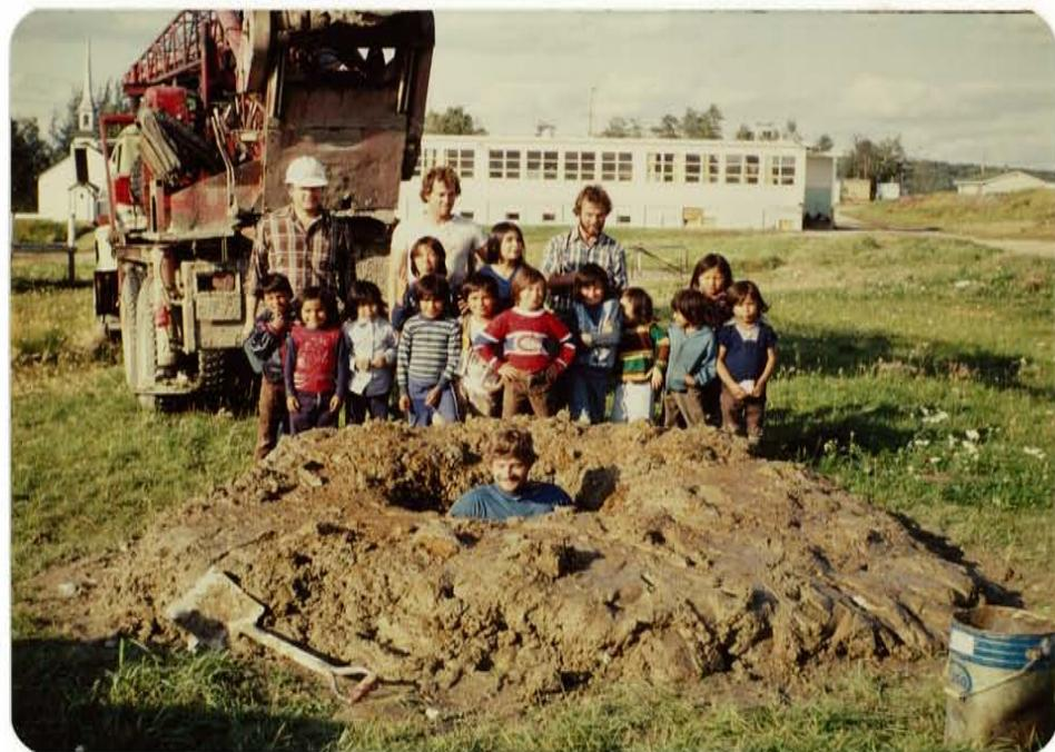
Figure 14. Augerhole site EAC-7 in which groundwater was encountered in the Lower Sand at a depth of 6.4 m.
