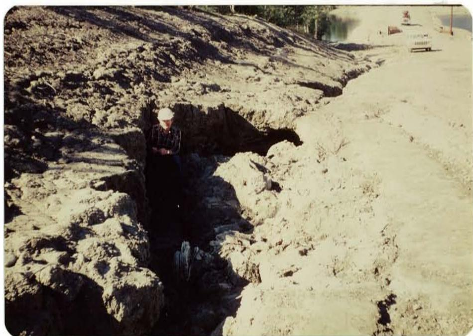
Figure 12. Gully erosion in ditch along Highway 102 between EAC - 13 and 14 (Drawing 0052-002-01). EAC - 13 is between bridge in causeway fill of channel and white truck.
