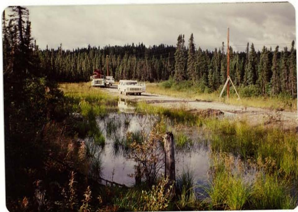
Figure 15. Runoff from surficial Silt and Clay and silty Till units and delayed runoff from the more permeable overlying Upper Gravel and Upper Sand units at EAC - 1 (Drawing 0052-002-01). Notice the upturned culvert caused by grade settlement in the boggy soils.
